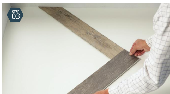
STEP 03 Install 2nd plank Take a second plank (B) and drop it with the long side engaging against the first plank (A) on the short side.
