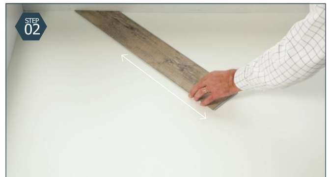
STEP 02 Install 1st plank Place the first plank (A) with the cut side against the wall at a 45° angle.
